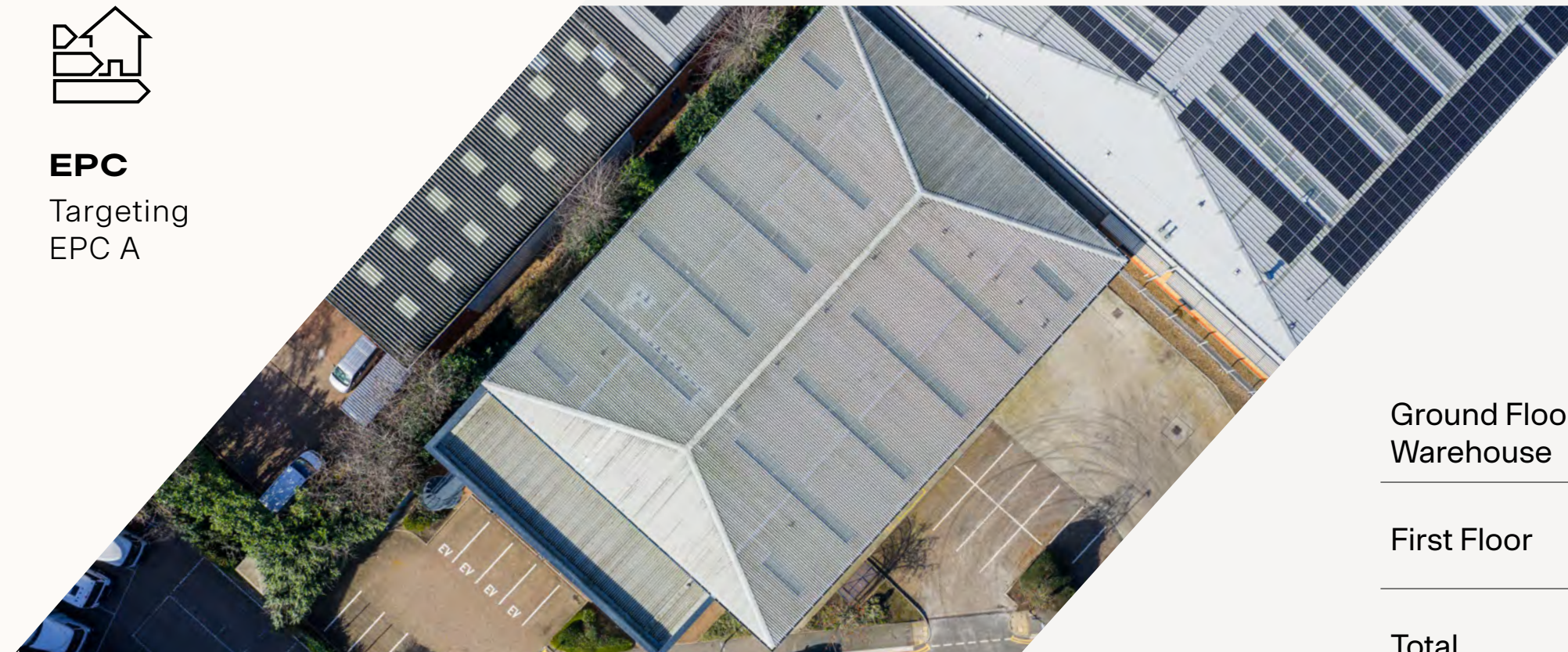
Unit 2 Aerial View
